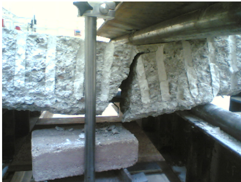
Figure 8: Cracking Pattern for One-layer Panel in Shear Test
