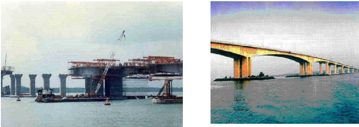
Fig. 2 Tuas bridge (a) under construction (b) under use
