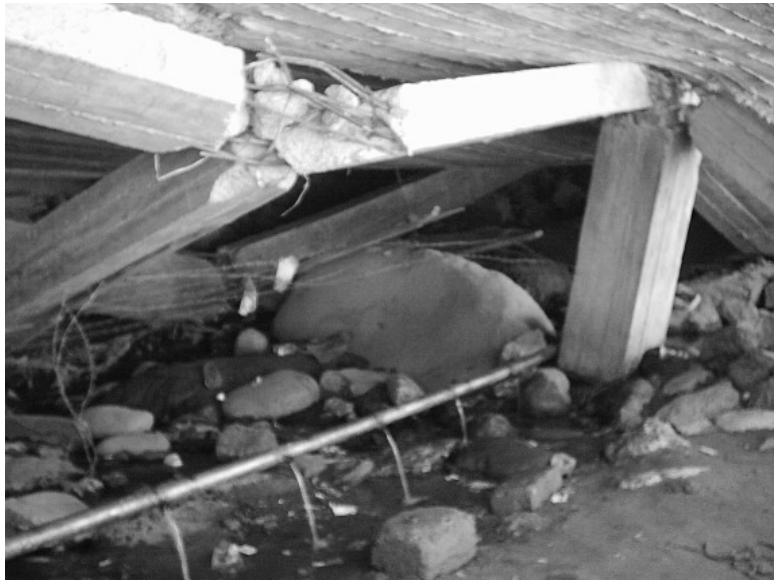
Figure 6: Frame Non-Monolith With Slab
