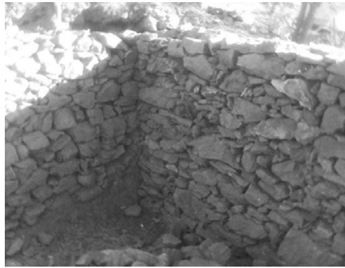
Figure 13: Un-Bonded Rubbles Being Dressed To Make A Load Bearing Wall Structure.
