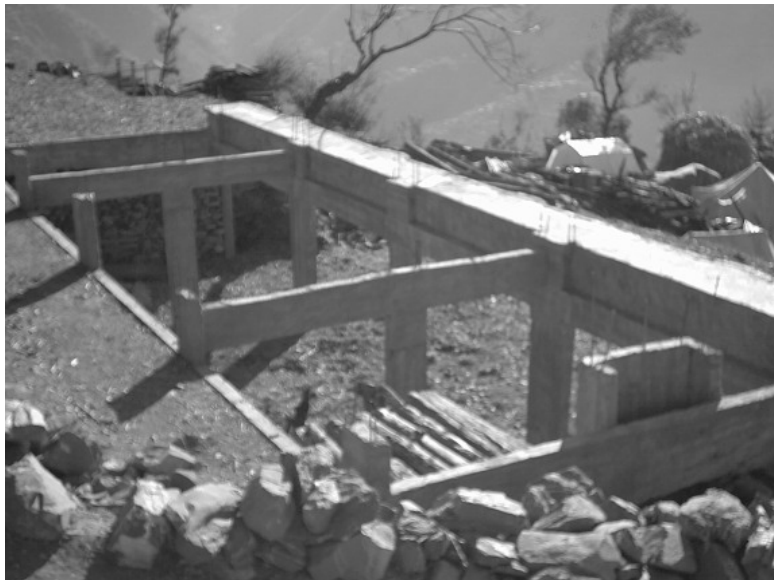
Figure 7: A Frame Structure In Pambara, Ready For Placing Slab.
