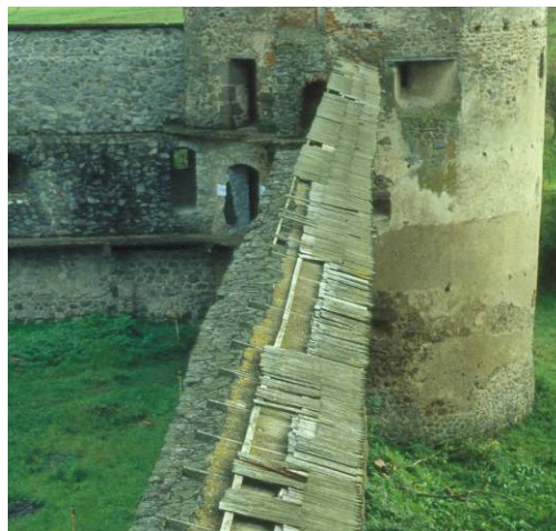
Figures 17, 18, 19: Three examples of newly built roof on fortifications – a reconstructed roof of a bastion of the town wall of Nürnberg (Germany, left), a very good example of a newly built roof on the tower of the castle of Stará Ľubovňa (Slovakia, right) and a largely damaged roof cover of the walls on a not maintained ruin of the fortified monastery of Bzovík (Slovakia, down).
