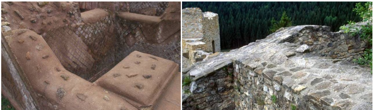
Figures 5, 6: Left - an example of the use of mortar filled with some pieces of brocks on the wall coping of roman walls at Ostia (Italy) – the whole shape of the coping looks generally a little bit strange. Right straightly shaped wall coping of the castle of Likava (Slovakia), with the use of flat stones placed into concrete – not natural deformation of the shape of the walls is mostly visible only from a near look.
