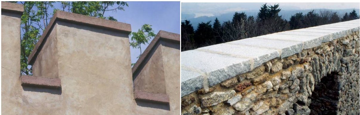
Figures 12, 13: Covers made from concrete (left – on the castle of Vígľaš in Slovakia) and from stone plates (right the castle of Vítkův hrádek in Czechia) – both are giving the ruin a slightly artificial appearance and also their protection role is a bit far from being perfect.
