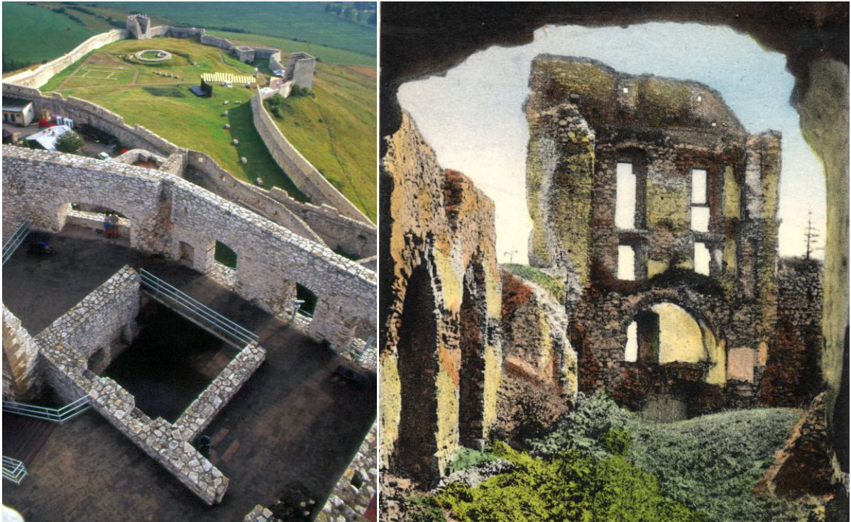
Figures 1, 2: Typical examples of wall copings of ruined architecture - left the castle of Spiš with not naturally looking straight line of copings (after the conservation) and the castle of Pajštún with natural curved copings of a “romantic appearance” (postcard, 19 th century) – both in Slovakia.
