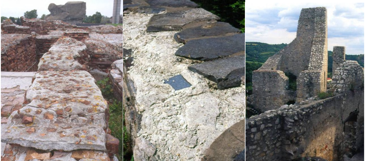
Figures 7, 8, 9: Examples of various technologies – use of lime mortar filled with pieces of bricks on the fortress of Brest (Belarus) does not protect the walls very much, as it mostly broke away already (left). Use of volcanic stone plates, placed into strong cement mortar did also not worked properly – castle of Vígľaš (Slovakia), 8 years after realization (center) and very artificially formed skyline of the ruin of Beckov by massive use of added stone masonry fitted by deep injection with expansive cement (right).
