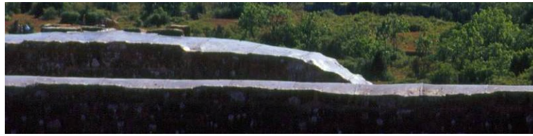
Figure 14: An example of use of tin plates for protection of walls (Borgholm castle, Öland, Sweden)
